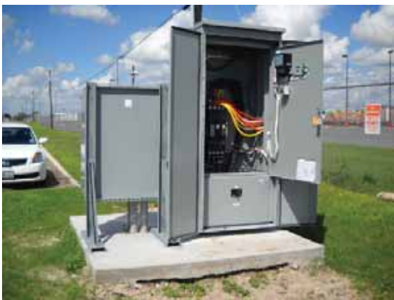
Inside wiring of an ATS
